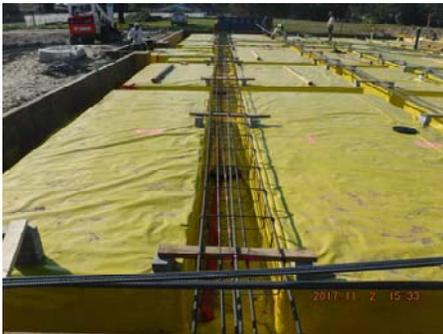
**FOUNDATION GRADE BEAMS WITH STRUCTURAL REINFORCEMENT — ADMINISTRATION BUILDING AND FRONT ENTRANCE**
