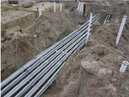
**ELECTRICAL AND COMMUNICATIONS CONDUIT BELOW FOUNDATION OF SAFEHOUSE BUILDING**
