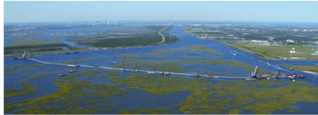
IHNC Surge Barrier
