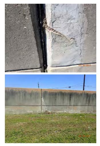
Inspect ID: USACE\_CEMVN\_OLD1\_2017\_a\_0022 Title: USACE\_CEMVN\_OLD1\_2017\_a\_0022\_3.jpg Rated Item: 04. Concrete Surfaces Rating: M Inspection Remarks: Numerous spalls along the landside of the floodwall. Recommended Action: SLFPA-E shall monitor concrete cracking/degradation and make corrective actions as required. Caption: Station 1: 67+13 (IHNCW) Station 2: 74+47 (IHNCW)
