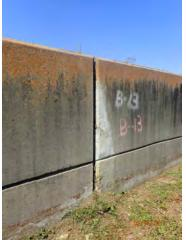
Inspect ID: USACE\_CEMVN\_OLD1\_2017\_a\_0022 Title: USACE\_CEMVN\_OLD1\_2017\_a\_0022\_1.jpg Rated Item: 04. Concrete Surfaces Rating: M Inspection Remarks: Numerous spalls along the landside of the floodwall. Recommended Action: SLFPA-E shall monitor concrete cracking/degradation and make corrective actions as required. Caption: Station 1: 67+13 (IHNCW) Station 2: 74+47 (IHNCW)
