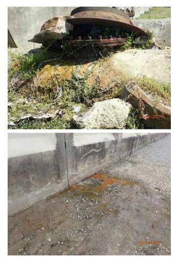
Inspect ID: USACE\_CEMVN\_OLD1\_2017\_a\_0011 Title: USACE\_CEMVN\_OLD1\_2017\_a\_0011\_1.jpg Rated Item: 02. Encroachments Rating: M Inspection Remarks: Leaking water pipe on the floodside. Recommended Action: SLFPA-E should coordinate with the Sewerage and Water Board to make corrective action. Caption: Station 1: 70+62 (IHNCW)
