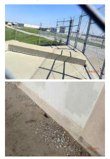
Inspect ID: USACE\_CEMVN\_OLD1\_2017\_a\_0021 Title: USACE\_CEMVN\_OLD1\_2017\_a\_0021\_1.jpg Rated Item: 06. Foundation of Concrete Structures Rating: M Inspection Remarks: Sealant deterioration at the floodwall and scour protection on the protected side. Recommended Action: SLFPA-E shall make corrective actions as required. Clean concrete surface. Seal cracks. Patch concrete. Seal concrete. Caption: Station 1: 430+09 (OP)
