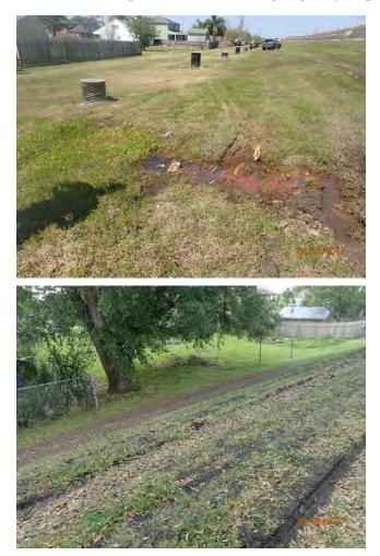
Inspect ID: USACE\_CEMVN\_OLD1\_2017\_a\_0015 Title: USACE\_CEMVN\_OLD1\_2017\_a\_0015\_2.jpg Rated Item: 08. Depressions/ Rutting Rating: M Inspection Remarks: Ruts with ponding water on landside of wall near relief well. Recommended Action: SLFPA-E shall repair depressed or rutted areas with compacted clay fill. The areas shall then be fertilized and seeded. Caption: Station 1: 253+37 (IHNCW)
