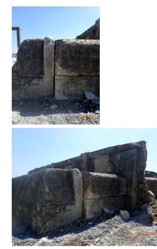
Inspect ID: USACE\_CEMVN\_OLD1\_2017\_a\_0006 Title: USACE\_CEMVN\_OLD1\_2017\_a\_0006\_2.jpg Rated Item: 07. Monolith Joints Rating: M Inspection Remarks: Water stop deterioration. Recommended Action: SLFPA-E needs to repair the expansion material between monolith joints. Caption: Station 1: 53+25 (IHNCW)
