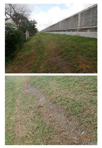
Inspect ID: USACE\_CEMVN\_OLD1\_2017\_a\_0108 Title: USACE\_CEMVN\_OLD1\_2017\_a\_0108\_1.jpg Rated Item: 08. Depressions/ Rutting Rating: M Inspection Remarks: Ruts along the landside levee slope. Recommended Action: SLFPA-E shall repair eroded areas with compacted clay fill. The areas shall then be fertilized and seeded. Caption: Station 1: 84+11 (LCE)
