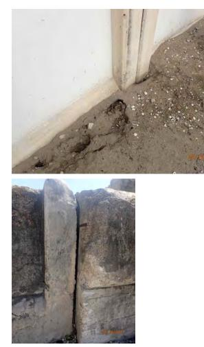
Inspect ID: USACE\_CEMVN\_OLD1\_2017\_a\_0023 Title: USACE\_CEMVN\_OLD1\_2017\_a\_0023\_4.jpg Rated Item: 06. Foundation of Concrete Structures Rating: Inspection Remarks: Small voids at the base of the floodwall on floodside. Recommended Action: SLFPA-E shall inspect, repair, and monitor damaged areas. Caption: Station 1: 474+34 (OLD)
