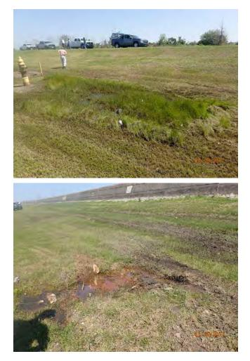
Inspect ID: USACE\_CEMVN\_OLD1\_2017\_a\_0005 Title: USACE\_CEMVN\_OLD1\_2017\_a\_0005\_3.jpg Rated Item: 08. Depressions/ Rutting Rating: M Inspection Remarks: Ponding water near fire hydrant on floodside. Recommended Action: SLFPA-E shall repair depressed or rutted areas with compacted clay fill. The areas shall then be fertilized and seeded. Caption: Station 1: 21+73 (IHNCW)
