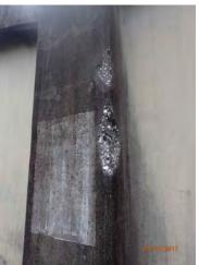
Inspect ID: USACE\_CEMVN\_OLD1\_2017\_a\_0022 Title: USACE\_CEMVN\_OLD1\_2017\_a\_0022\_5.jpg Rated Item: 04. Concrete Surfaces Rating: M Inspection Remarks: Numerous spalls along the landside of the floodwall. Recommended Action: SLFPA-E shall monitor concrete cracking/degradation and make corrective actions as required. Caption: Station 1: 67+13 (IHNCW) Station 2: 74+47 (IHNCW)
