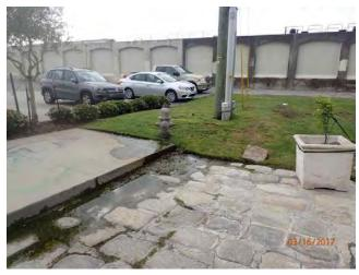
Inspect ID: USACE\_CEMVN\_OLD1\_2017\_a\_0024 Title: USACE\_CEMVN\_OLD1\_2017\_a\_0024\_4.jpg Rated Item: 02. Encroachments Rating: M Inspection Remarks: Leaking fire hydrant causing ponding water at the base of floodwall. Recommended Action: SLFPA-E should coordinate with the Sewerage and Water Board to make corrective action. Caption: Station 1: 534+82 (OLD)
