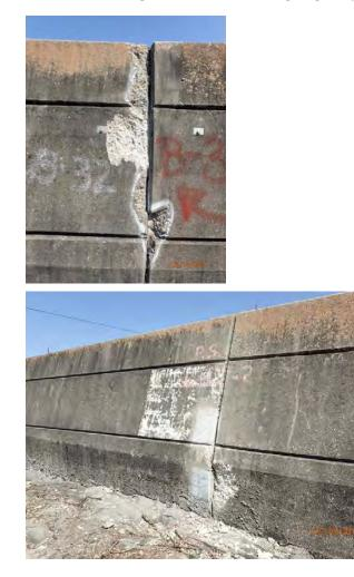
Inspect ID: USACE\_CEMVN\_OLD1\_2017\_a\_0016 Title: USACE\_CEMVN\_OLD1\_2017\_a\_0016\_1.jpg Rated Item: 04. Concrete Surfaces Rating: M Inspection Remarks: Spall along joint of floodwall. Recommended Action: SLFPA-E shall monitor concrete cracking/degradation and make corrective actions as required. Caption: Station 1: 263+13 (IHNCW)
