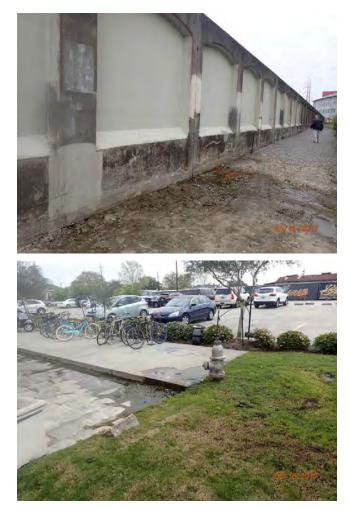
Inspect ID: USACE\_CEMVN\_OLD1\_2017\_a\_0024 Title: USACE\_CEMVN\_OLD1\_2017\_a\_0024\_2.jpg Rated Item: 02. Encroachments Rating: M Inspection Remarks: Leaking fire hydrant causing ponding water at the base of floodwall. Recommended Action: SLFPA-E should coordinate with the Sewerage and Water Board to make corrective action. Caption: Station 1: 534+82 (OLD)
