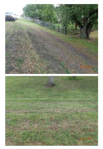
Inspect ID: USACE\_CEMVN\_OLD1\_2017\_a\_0101 Title: USACE\_CEMVN\_OLD1\_2017\_a\_0101\_2.jpg Rated Item: 08. Depressions/ Rutting Rating: M Inspection Remarks: Rutting and erosion on the landside levee slope below the floodwall. Recommended Action: SLFPA-E shall repair depressed or rutted areas with compacted clay fill. The areas shall then be fertilized and seeded. SLFPA-E has a contract out for this to be repaired. Caption: Station 1: 587+14 (17E)
