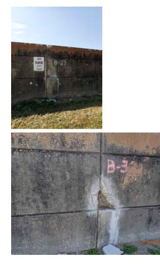
Inspect ID: USACE\_CEMVN\_OLD1\_2017\_a\_0017 Title: USACE\_CEMVN\_OLD1\_2017\_a\_0017\_1.jpg Rated Item: 04. Concrete Surfaces Rating: M Inspection Remarks: Previously repaired spall but deteriorating again. Recommended Action: SLFPA-E shall monitor concrete cracking/degradation and make corrective actions as required. Caption: Station 1: 247+84 (IHNCW)
