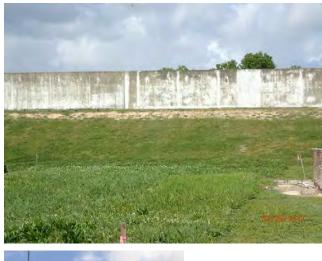
Inspect ID: USACE\_CEMVN\_OLD1\_2017\_a\_0110 Title: USACE\_CEMVN\_OLD1\_2017\_a\_0110\_1.jpg Rated Item: 02. Sod Cover Rating: M Inspection Remarks: Lack of sod cover along crown. SLFPA-E has plans to repair. Recommended Action: SLFPA-E shall fertilize and seed areas until adequate sod cover is achieved. Caption: Station 1: 116+19 (LCE)
