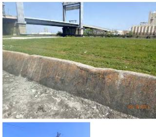
Inspect ID: USACE\_CEMVN\_OLD1\_2017\_a\_0012 Title: USACE\_CEMVN\_OLD1\_2017\_a\_0012\_1.jpg Rated Item: 04. Concrete Surfaces Rating: M Inspection Remarks: Spalling at top of wall. Recommended Action: SLFPA-E shall monitor concrete cracking/degradation and make corrective actions as required. Caption: Station 1: 189+78 (IHNCW)
