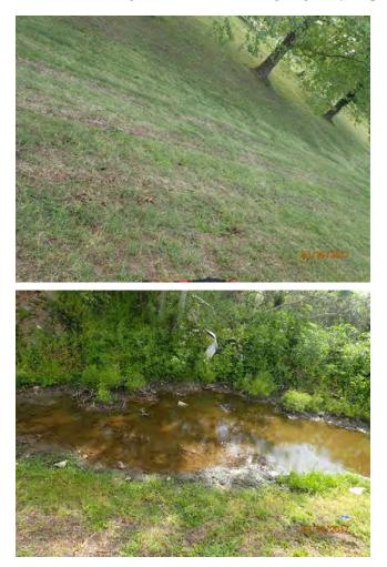
Inspect ID: USACE\_CEMVN\_OLD1\_2017\_a\_0105 Title: USACE\_CEMVN\_OLD1\_2017\_a\_0105\_2.jpg Rated Item: 08. Depressions/ Rutting Rating: M Inspection Remarks: Depressions from mowers. Recommended Action: SLFPA-E shall repair depressed or rutted areas with compacted clay fill. The areas shall then be fertilized and seeded. Caption: Station 1: 15+33 (OCE)
