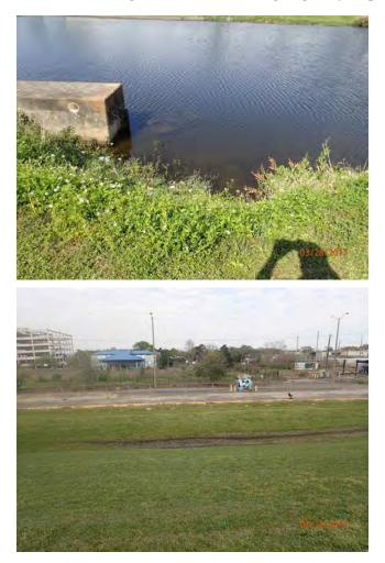
Inspect ID: USACE\_CEMVN\_OLD1\_2017\_a\_0102 Title: USACE\_CEMVN\_OLD1\_2017\_a\_0102\_1.jpg Rated Item: 06. Erosion/ Bank Caving Rating: M Inspection Remarks: Erosion around southeast end of the 17th Street Outfall Canal pump station wingwall. Recommended Action: SLFPA-E should monitor the erosion and contact USACE if conditions worsen. Caption: Station 1: 669+93 (17E)
