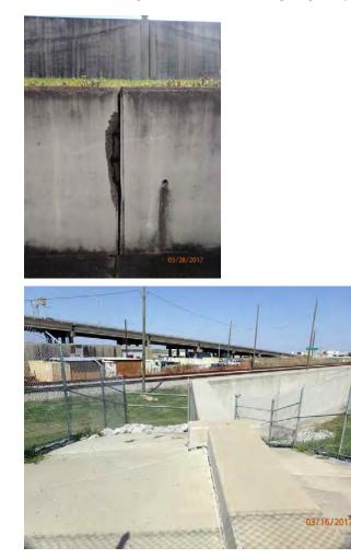
Inspect ID: USACE\_CEMVN\_OLD1\_2017\_a\_0103 Title: USACE\_CEMVN\_OLD1\_2017\_a\_0103\_1.jpg Rated Item: 04. Concrete Surfaces Rating: M Inspection Remarks: Exposed rebar on the landside retaining wall below the floodwall at Orleans Canal. Recommended Action: SLFPA-E shall make corrective actions as required. Caption: Station 1: 77+28 (OCW) Station 2: 84+06 (OCW)
