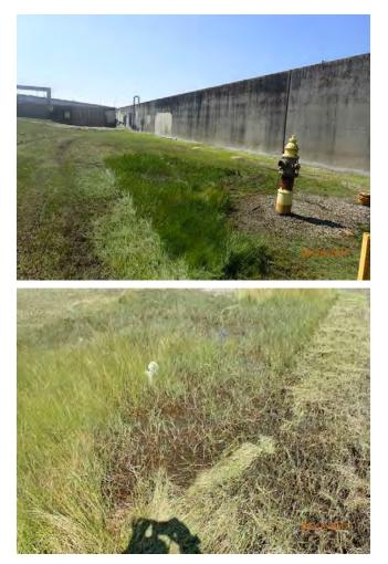
Inspect ID: USACE\_CEMVN\_OLD1\_2017\_a\_0005 Title: USACE\_CEMVN\_OLD1\_2017\_a\_0005\_1.jpg Rated Item: 08. Depressions/ Rutting Rating: M Inspection Remarks: Ponding water near fire hydrant on floodside. Recommended Action: SLFPA-E shall repair depressed or rutted areas with compacted clay fill. The areas shall then be fertilized and seeded. Caption: Station 1: 21+73 (IHNCW)
