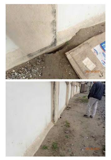
Inspect ID: USACE\_CEMVN\_OLD1\_2017\_a\_0023 Title: USACE\_CEMVN\_OLD1\_2017\_a\_0023\_2.jpg Rated Item: 06. Foundation of Concrete Structures Rating: Inspection Remarks: Small voids at the base of the floodwall on floodside. Recommended Action: SLFPA-E shall inspect, repair, and monitor damaged areas. Caption: Station 1: 474+34 (OLD)
