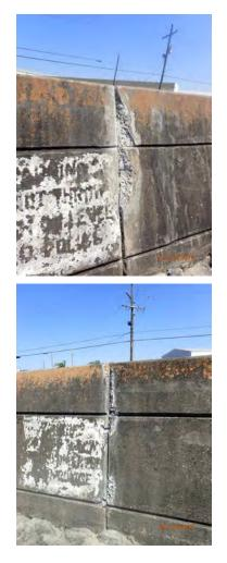
Inspect ID: USACE\_CEMVN\_OLD1\_2017\_a\_0014 Title: USACE\_CEMVN\_OLD1\_2017\_a\_0014\_1.jpg Rated Item: 04. Concrete Surfaces Rating: M Inspection Remarks: Spall along joint of floodwall. Recommended Action: SLFPA-E shall monitor concrete cracking/degradation and make corrective actions as required. Caption: Station 1: 251+76 (IHNCW)
