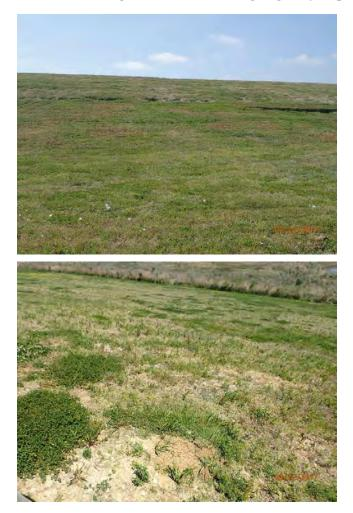
Inspect ID: USACE\_CEMVN\_OLD2\_2017\_a\_0006 Title: USACE\_CEMVN\_OLD2\_2017\_a\_0006\_1.jpg Rated Item: 02. Sod Cover Rating: M Inspection Remarks: Poor sod cover on slope leading to some erosion. Recommended Action: SFLPA-E shall fertilize and seed areas until adequate sod cover is achieved. Caption: Station 1: 336+05 (NOECB) Station 2: 346+29 (NOECB)
