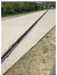
Inspect ID: USACE\_CEMVN\_OLD2\_2017\_a\_0004 Title: USACE\_CEMVN\_OLD2\_2017\_a\_0004\_1.jpg Rated Item: 06. Erosion/ Bank Caving Rating: M Inspection Remarks: Erosion on floodside slope Recommended Action: SFLPA-E should monitor erosion. Caption: Station 1: 321+53 (NOECB) Station 2: 324+47 (NOECB)
