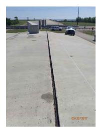
Inspect ID: USACE\_CEMVN\_OLD2\_2017\_a\_0014 Title: USACE\_CEMVN\_OLD2\_2017\_a\_0014\_1.jpg Rated Item: 13. Revetments other than Riprap Rating: A Inspection Remarks: Separation of splash pad. Recommended Action: SFLPA-E has filled gap and they should continue to monitor and make repairs in accordance with Vol. 2 of OMRR&R manual. Caption: Station 1: 939+41 (NOE)
