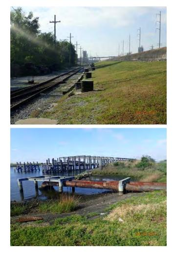
Inspect ID: USACE\_CEMVN\_OLD2\_2017\_a\_0001 Title: USACE\_CEMVN\_OLD2\_2017\_a\_0001\_1.jpg Rated Item: 06. Erosion/ Bank Caving Rating: M Inspection Remarks: Erosion on landside slope. Recommended Action: USACE Project Management is coordinating with SFLPA-E to repair erosion in this area. Caption: Station 1: 39+05 (IHNCNE) Station 2: 50+82 (IHNCNE)
