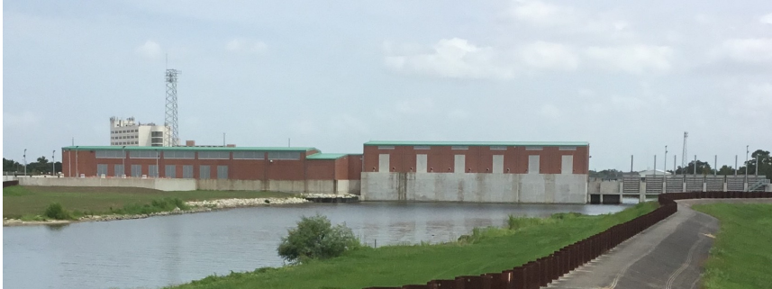
Permanent Canal Closure and Pumps at London Avenue
