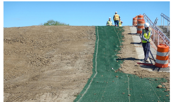
Top: Levee Maintenance Crew Bottom: Levee Armoring
