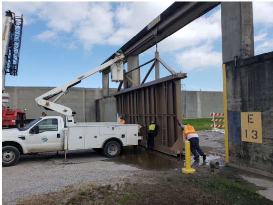
Crews close Floodgate S-01 (above) at Southern Scrap along the Industrial Canal and Floodgate E-13 (below)
