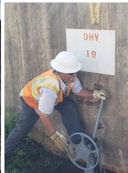
Closing valves (above and below)
