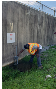
Closing valves (above and below)
