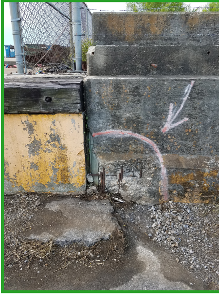
1. Before - Concrete damaged and old rebar exposed
