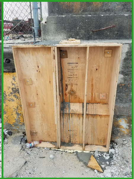
3. Form put in place and new concrete poured
