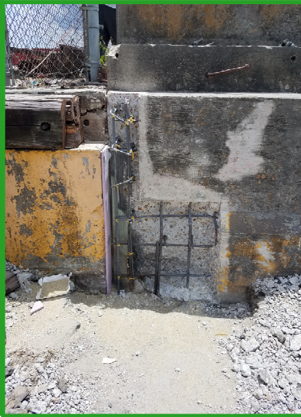
2. Pieces of old concrete chipped out; old rebar removed and replaced with new rebar
