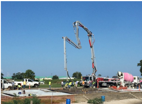
Contractor pouring slabs behind seawall at Seabrook (left).
