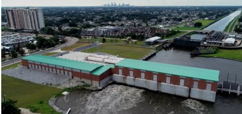
17th Street Outfall Canal—Permanent Canal Closure and Pumps in forefront and Interim Closure Structure and Temporary Pumps in rear
