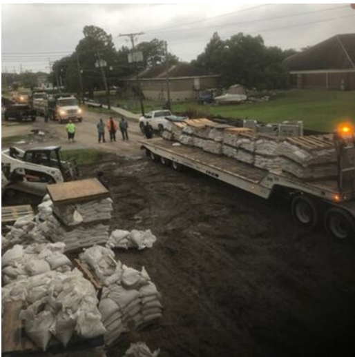
Sandbags being delivered to Lafitte, LA
