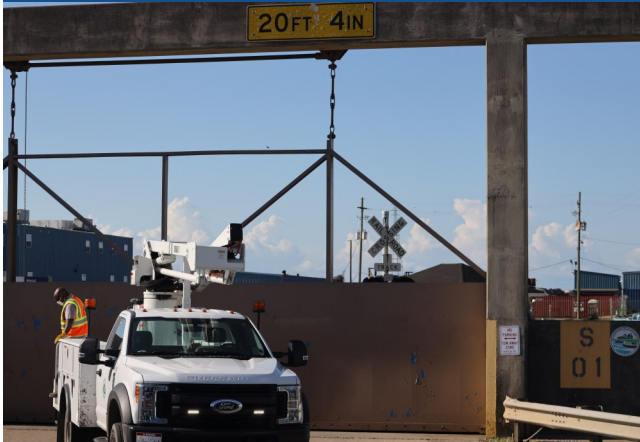
Maintenance crews close floodgates in advance of TS Cristobal
