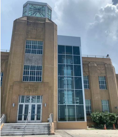
The new elevator constructed adjacent to the historic Terminal
