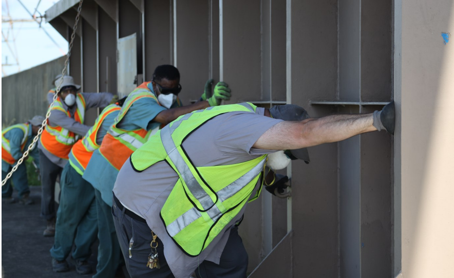
Floodgate closure in preparation for Tropical Storm Cristobal
