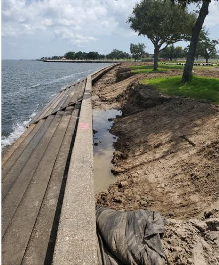
Soil removed behind seawall steps in order to make joint repairs prior to back-filling and driving vinyl sheet piles
