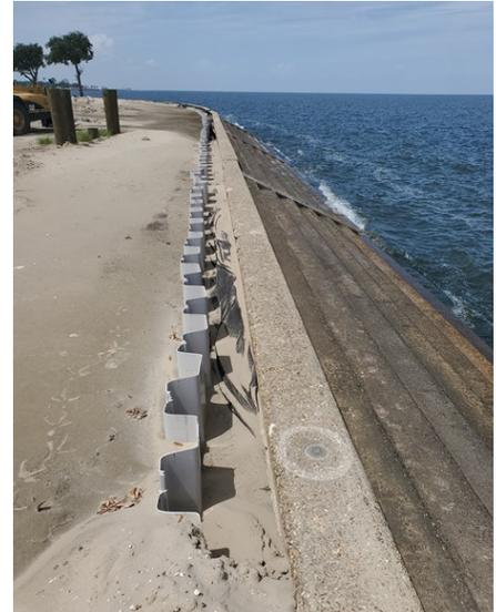
Vinyl sheet pile driven to prevent erosion
