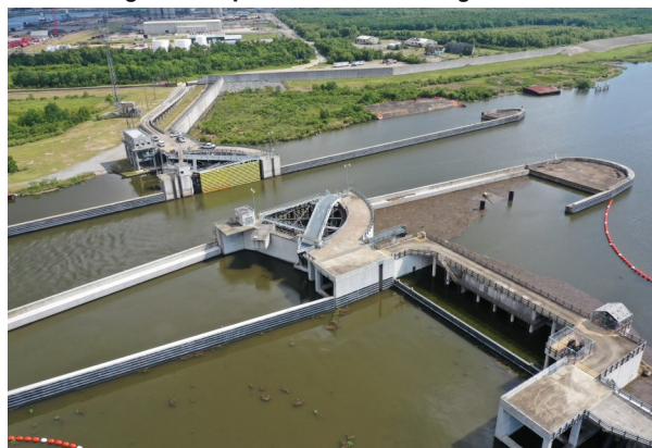
IHNC Surge Barrier Sector Gate and Barge Gate. Above with Barge Gate open; below with Barge Gate closed.
