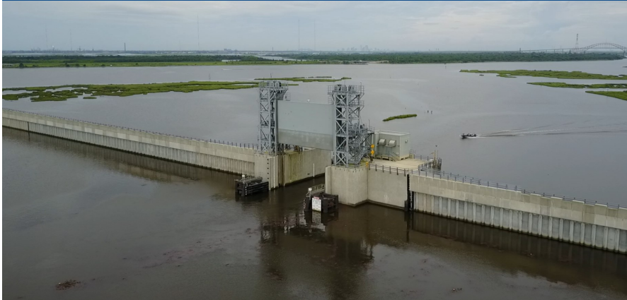
Bayou Bienvenue Vertical Lift Gate located in the IHNC Surge Barrier
