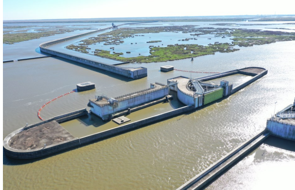
IHNC Surge Barrier Sector Gate and Barge Gate. Above with Barge Gate open; below with Barge Gate closed.
