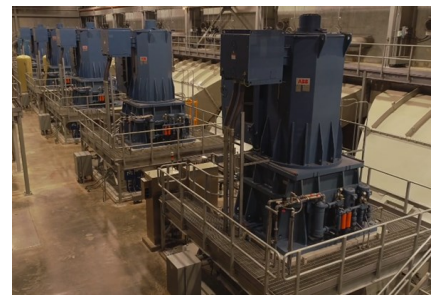
PCCP pumps (above) & generators (below)
