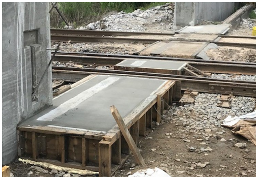
Left: Sill Placement, June 22, 2021
