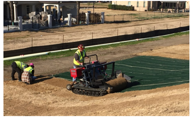
Levee Armoring with Turf Reinforced Matting
