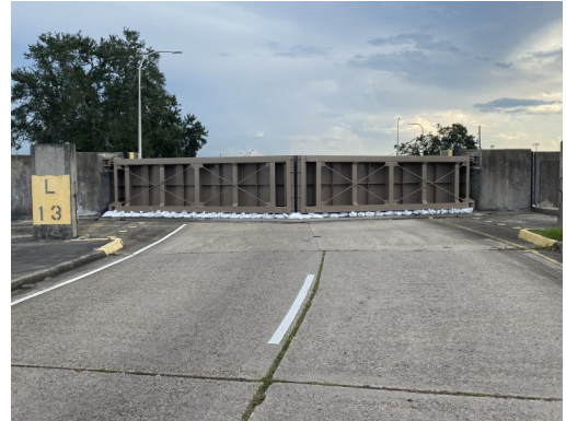
Floodgate L-13 at Lakeshore Drive west of Seabrook closed for Hurricane Ida
