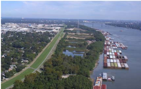
Mississippi River Levee
