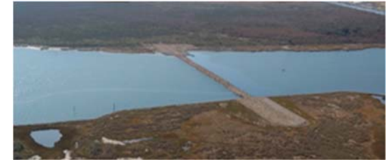
MR-GO Rock Dam Channel Closure
