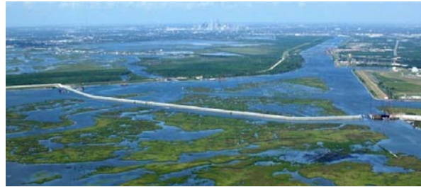
IHNC-Lake Borgne Surge Barrier
