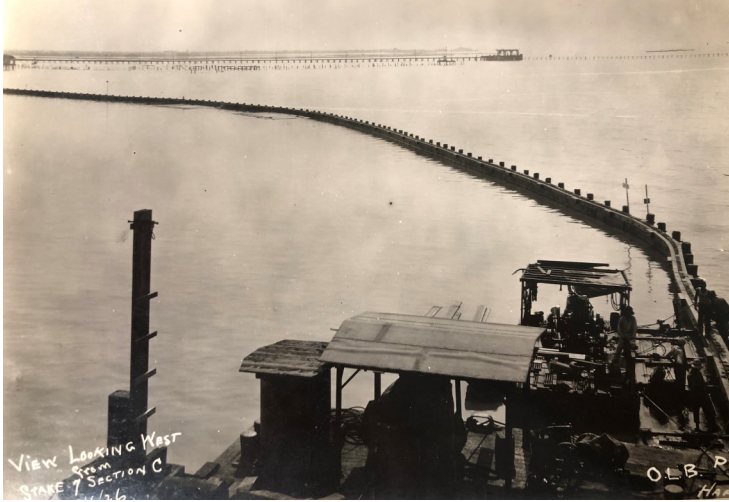
Pictured above Temporary Wooden Bulkhead
