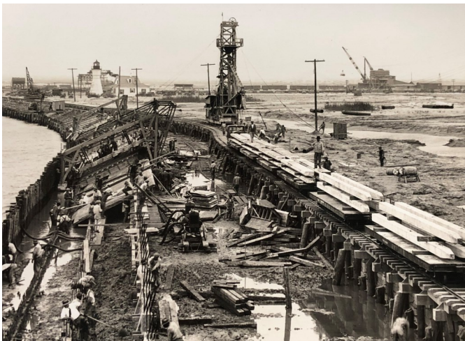
Construction of New Orleans Lakefront Seawall (1930-1932) stretching from the New Basin Canal to the Industrial Canal
