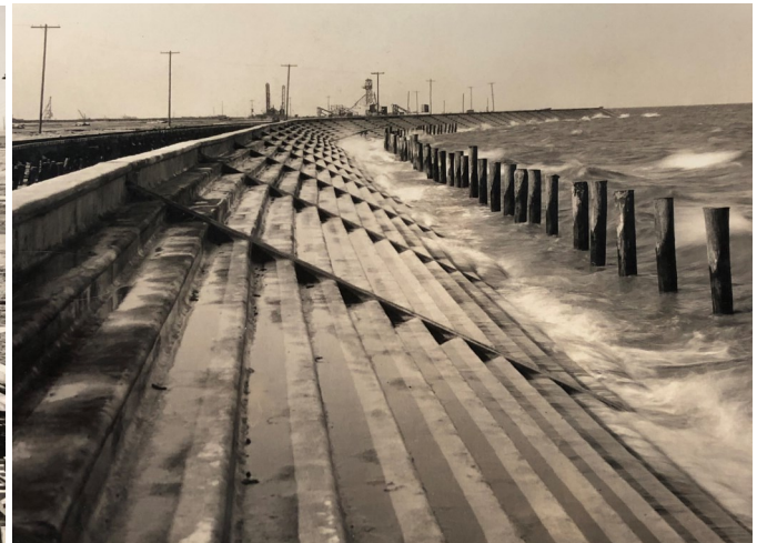
Construction of New Orleans Lakefront Seawall (1930-1932) stretching from the New Basin Canal to the Industrial Canal
