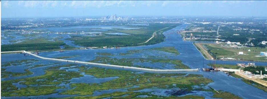
IHNC-Lake Borgne Surge Barrier
