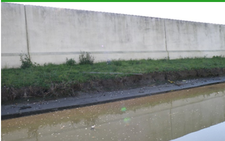
Pre-construction Condition Example
