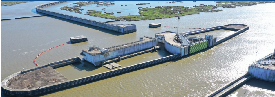
IHNC-Lake Borgne Surge Barrier Sector and Barge Gates
