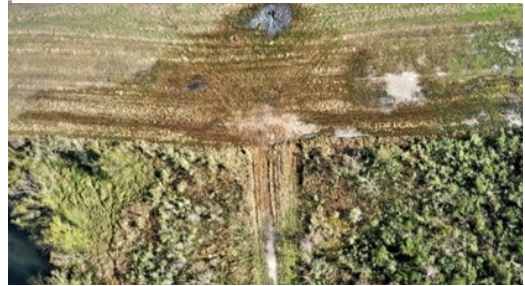
Pipeline Rupture and Spill Area East of Swing Bridge
