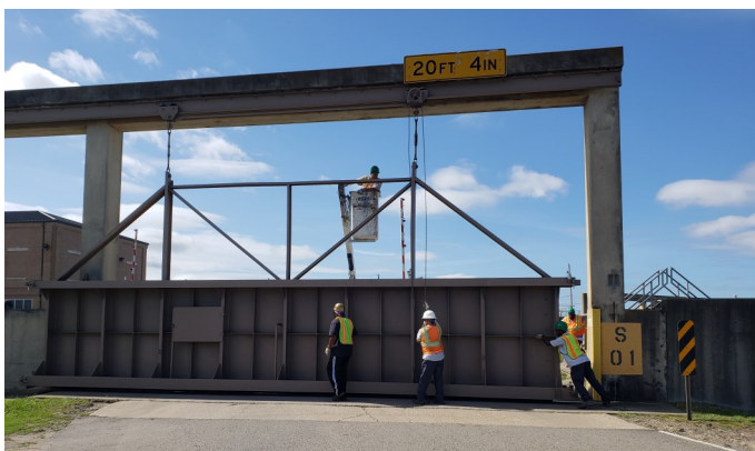
Crew closing Overhead Floodgate along MRGO
